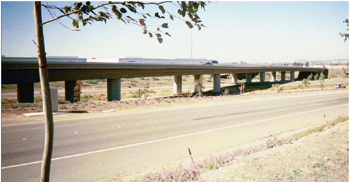
Northbound Jamboree Road Overcrossing, Orange County, California (Designed by Thomas Young, P.E.). This cast-in-place, pre-stressed, concrete box girder highway structure is located at the western end (post mile 0.0) of Highway 261. This was a FAST-TRACK, DESIGN/BUILD project.
